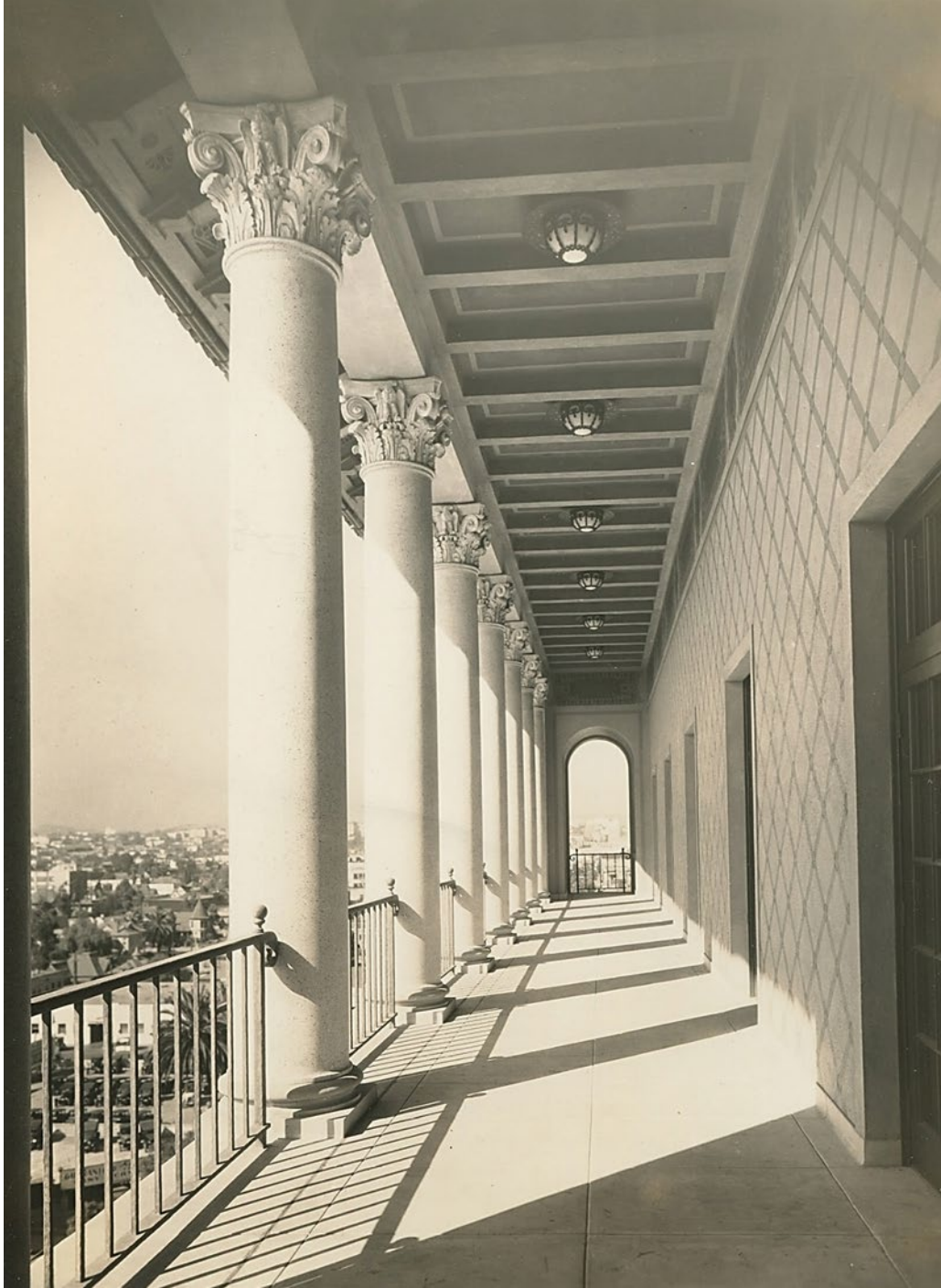
Figure 10 Loggia, eighth floor, leading from Admiral Chester H. Nimitz Room, 1926, facing north, DMVA, Bob Hope Patriotic Hall Archives
